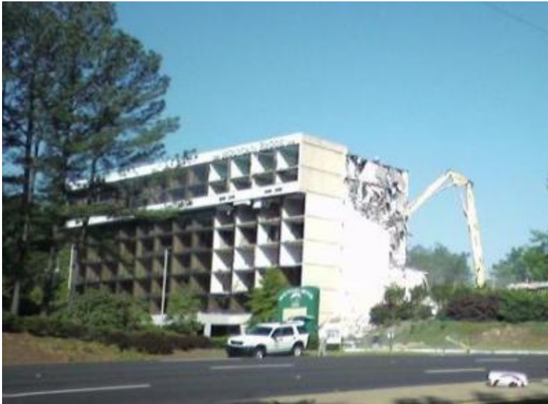
Mountain Brook Inn being demolished today. leadingzero /twitpic
